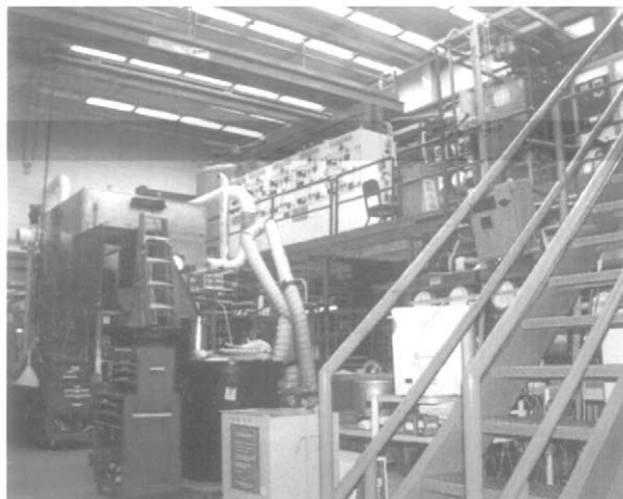
Fig. 4. North-looking view of TSTA test cell.
