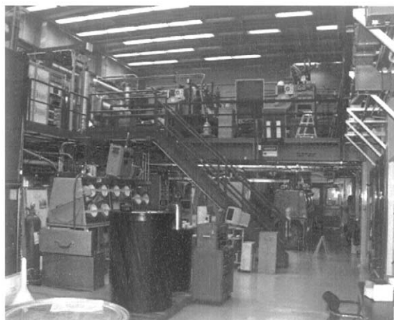
Fig. 3. South-looking view of TSTA test cell.
